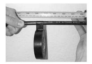
Figure 21 - Measure and mark the sheath opening at equal lengths from the reversal point.
