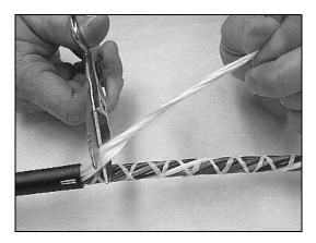
Figure 19 - Cut and remove the dielectric strength elements.
