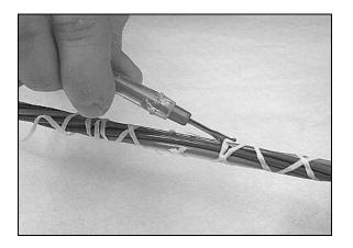
Figure 26 - Cut and remove the binder thread from the core.
