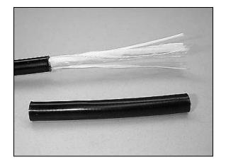
Figure 5 - Remove the 5-inch section of cable jacket.
