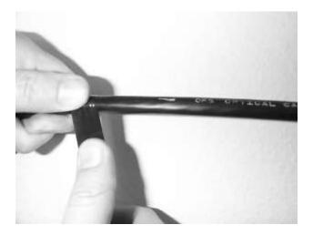
Figure 13 – Mark cable jacket with electrical tape.
