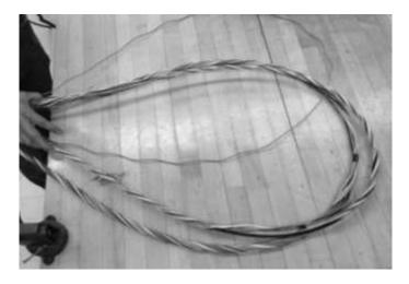
Figure 36 – Unwind the buffer tube(s) as far as possible as towards the end of the jacket opening.
