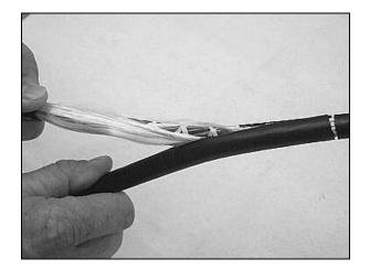
Figure 17 - Remove the 10-inch section of cable jacket.
