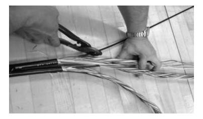
Figure 40 – Cut the central strength member to length as required for clamping in the closure.
