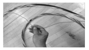
Figure 35 – Unwind the buffer tube(s) that will be routed to the splice tray.
