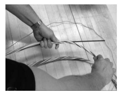
Figure 39 – Cut the central strength member in multiple steps while unwinding the buffer tubes.
