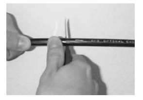
Figure 2 – Ring cut the cable sheath.
