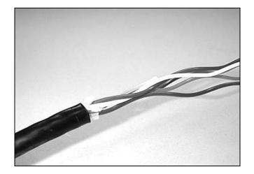
Figure 10 - Unwrap the buffer tubes.
