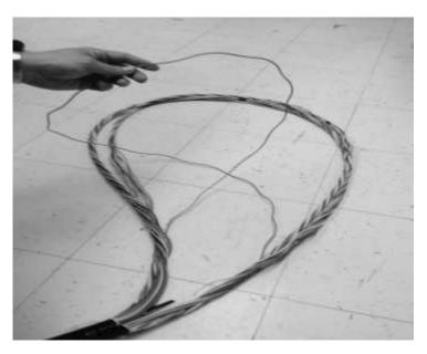
Figure 41 – Completed mid-span access of dual-layer cable.
