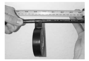
Figure 1 - Measure and mark the cable.
