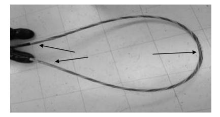
Figure 32 – Remove about 96" of cable jacket to expose three ROL locations indicated by the arrows.
