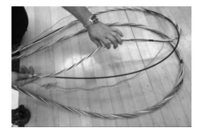
Figure 38 – Unwind the inner layer of buffer tubes to expose the central strength member.
