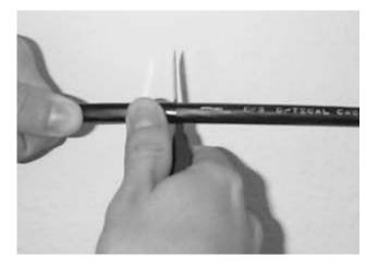
Figure 22 – Ring cut the cable jacket.
