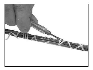
Figure 9 – Cut and remove binder threads.
