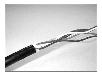
Figure 27 – Separate the buffer tubes. Page 13 of 20
