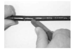
Figure 4 - Make a 5-inch longitudinal cut at the end of the cable.
