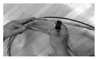
Figure 37 – Wrap a length of vinyl tape around the tubes at the ROL location.
